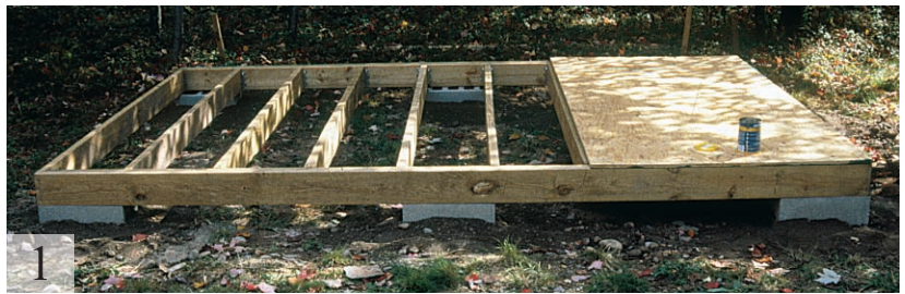
1 Prepare the site; then build the floor frame and position it on concrete blocks. Use only pressure-treated lumber and galvanized hangers and fasteners.
