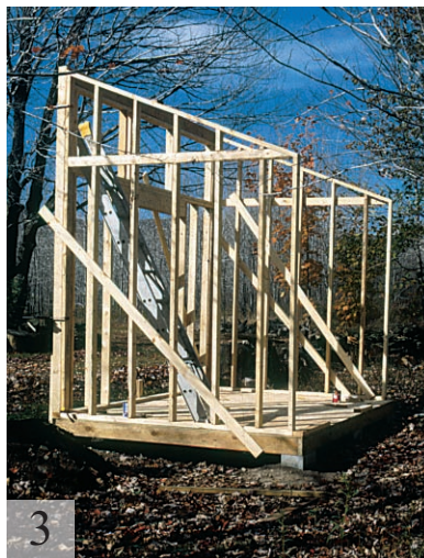
3 Erect the side walls and brace them with 2x4s. Nail 2x4 spacers to the floor to establish the rear wall position.
